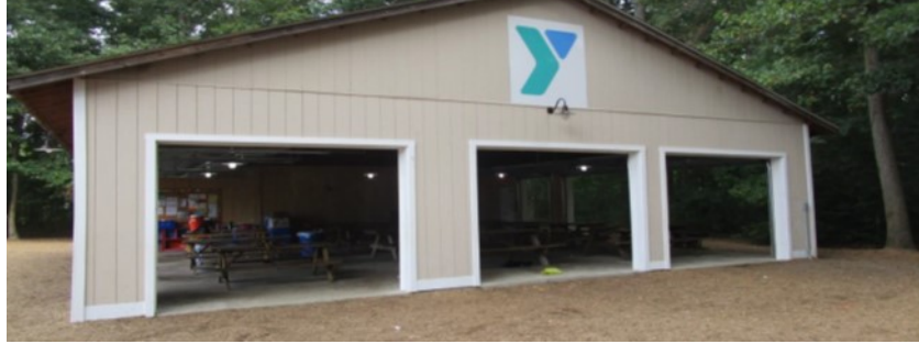
YMCA- Pavilion Renovation - 825 Kenton Road
