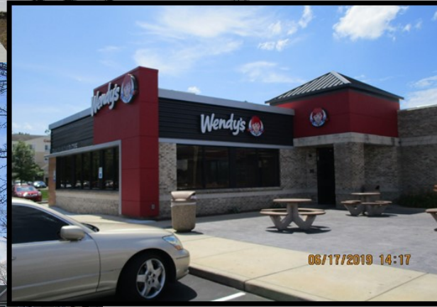
Wendy's Renovation—1710 N. DuPont Highway
