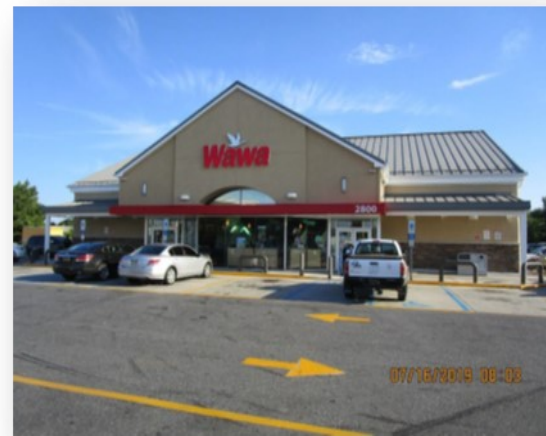
Renovations-2800 N DuPont Highway
